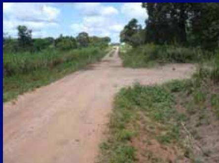
**...can cause side drains to overtop and erode the surface**
